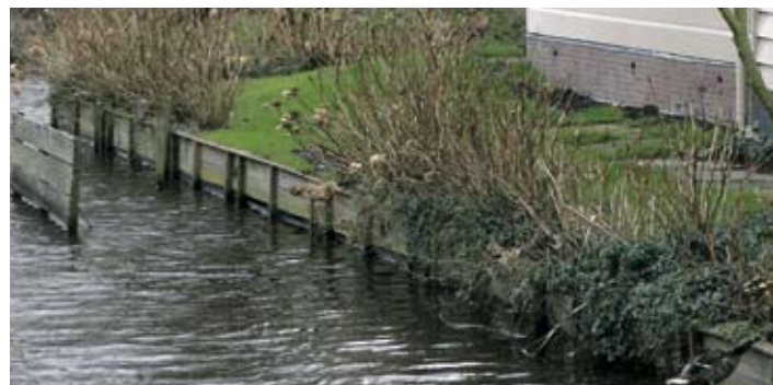
Houten beschoeiing, Broek in Waterland
